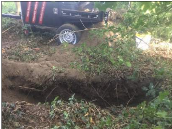
Foto 14: Sleuf SL12 (d.d. 21 september 2020)
