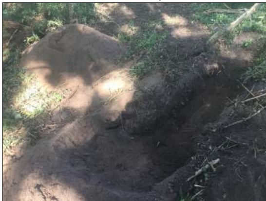
Foto 11: Sleuf SL09 (d.d. 21 september 2020)
